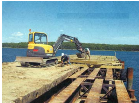
Category B City of Bath Southend Park Improvement Project
