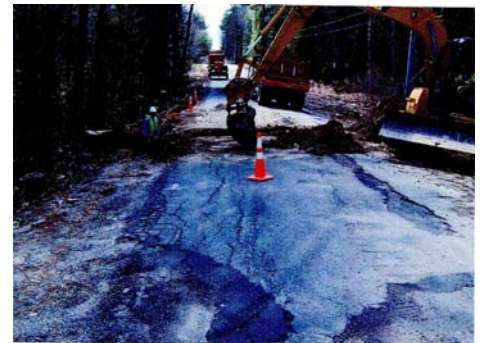
Category C Town of Pownal Allen Rd. Reconstruction Project
